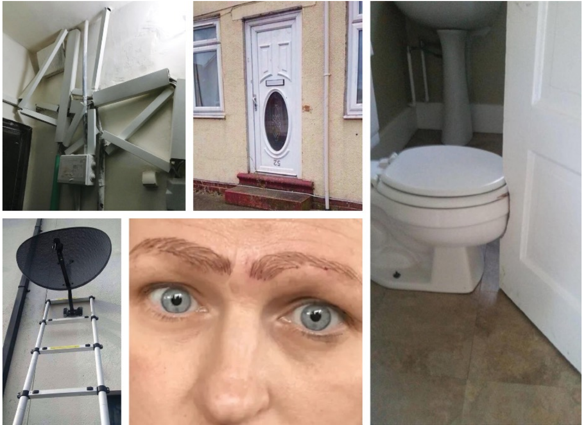
Figure 2.xix. (Top left) Cable conduit deployed in a wildly incorrect manner; (top centre) a front door fitted upside down; (right) a toilet installed before the critical ‘door test’ — the workaround being to remove part of the door to allow it to pass the toilet (the hole will likely impact privacy when the door is shut; (bottom left) a satellite dish installed through a ladder, instead of above it; (bottom centre) eyebrows haphazardly applied with a microblade device.
